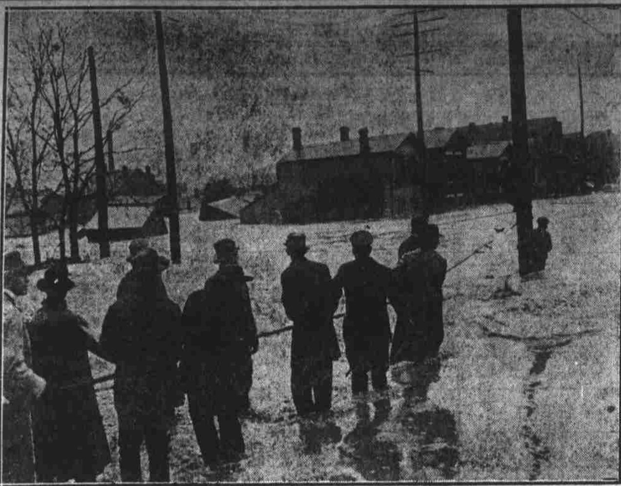
Tow lines wound about telegraph poles were used to hold boats engaged in rescue work from the flood current, which, running twenty miles an hour, made rowing impossible.
