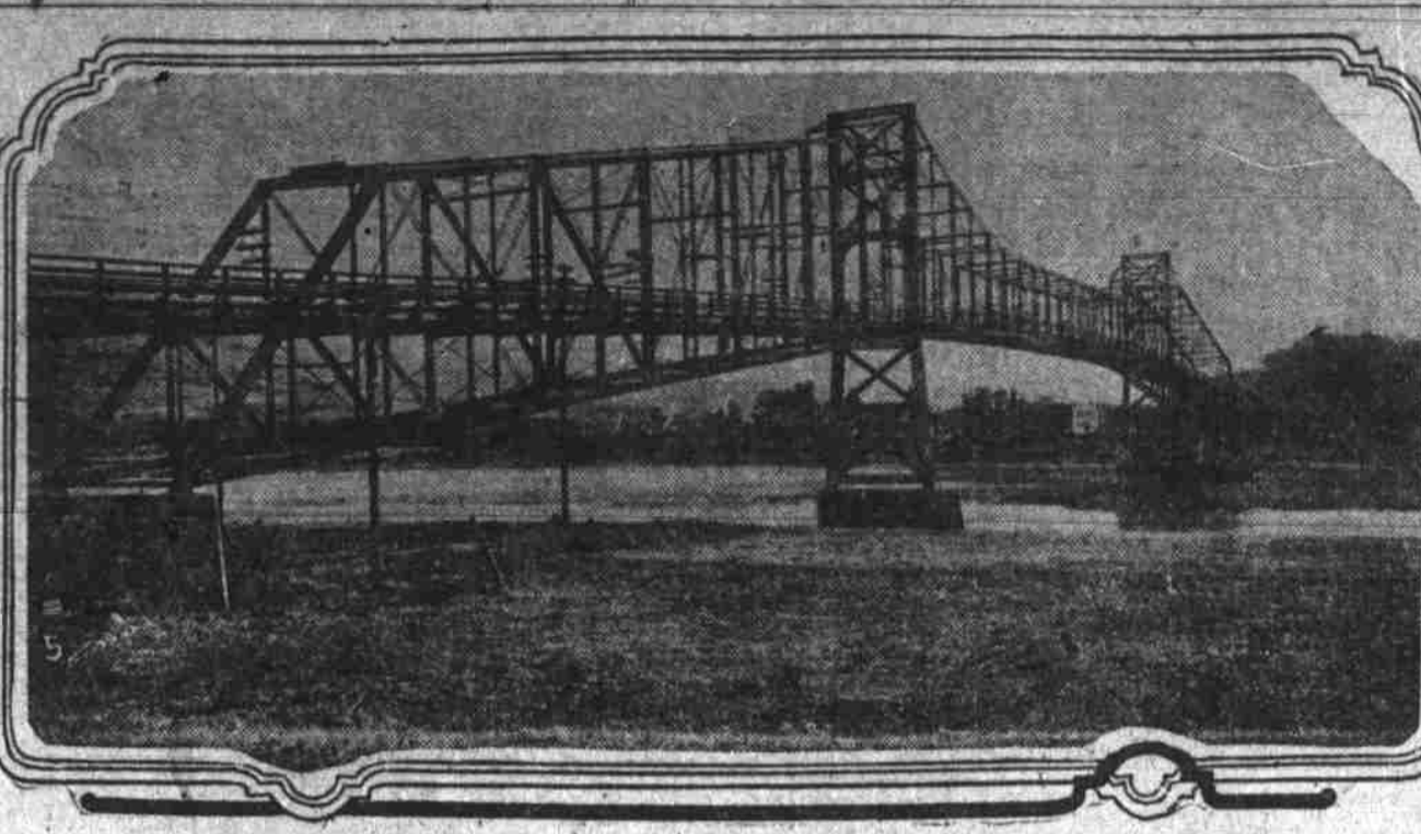
Washington-Idaho bridge across Snake river at Clarkston, Wash., bill for purchase of which has passed legislatures of two states.
