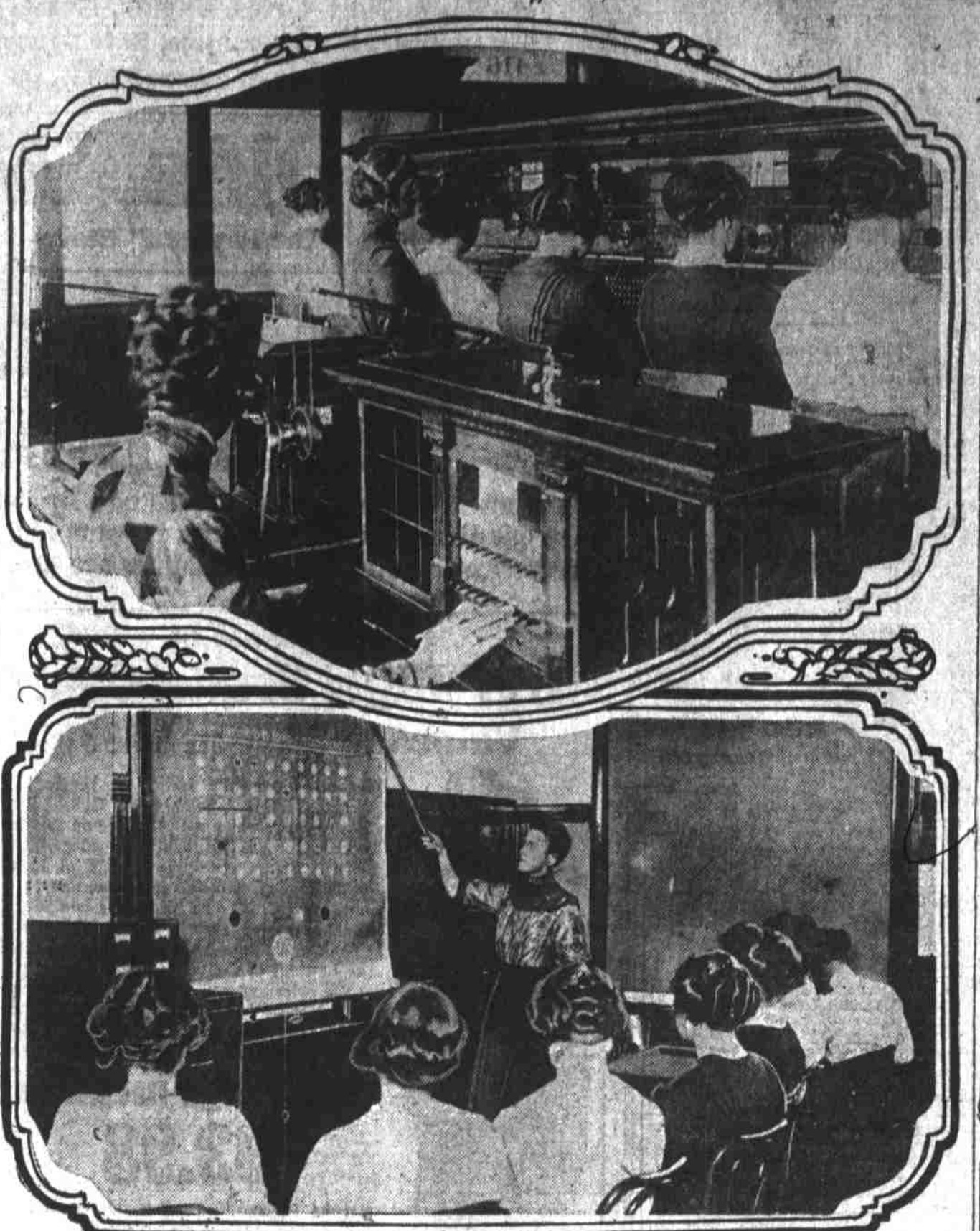
Student operators working a practice switchboard, at top. Group of girls receiving classroom instruction.
