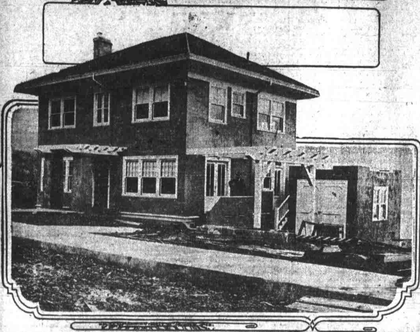
New residences at Westover Terraces. Top—Home of D. B. Hanson. Bottom—Residence of R. C. Hurlbert.
