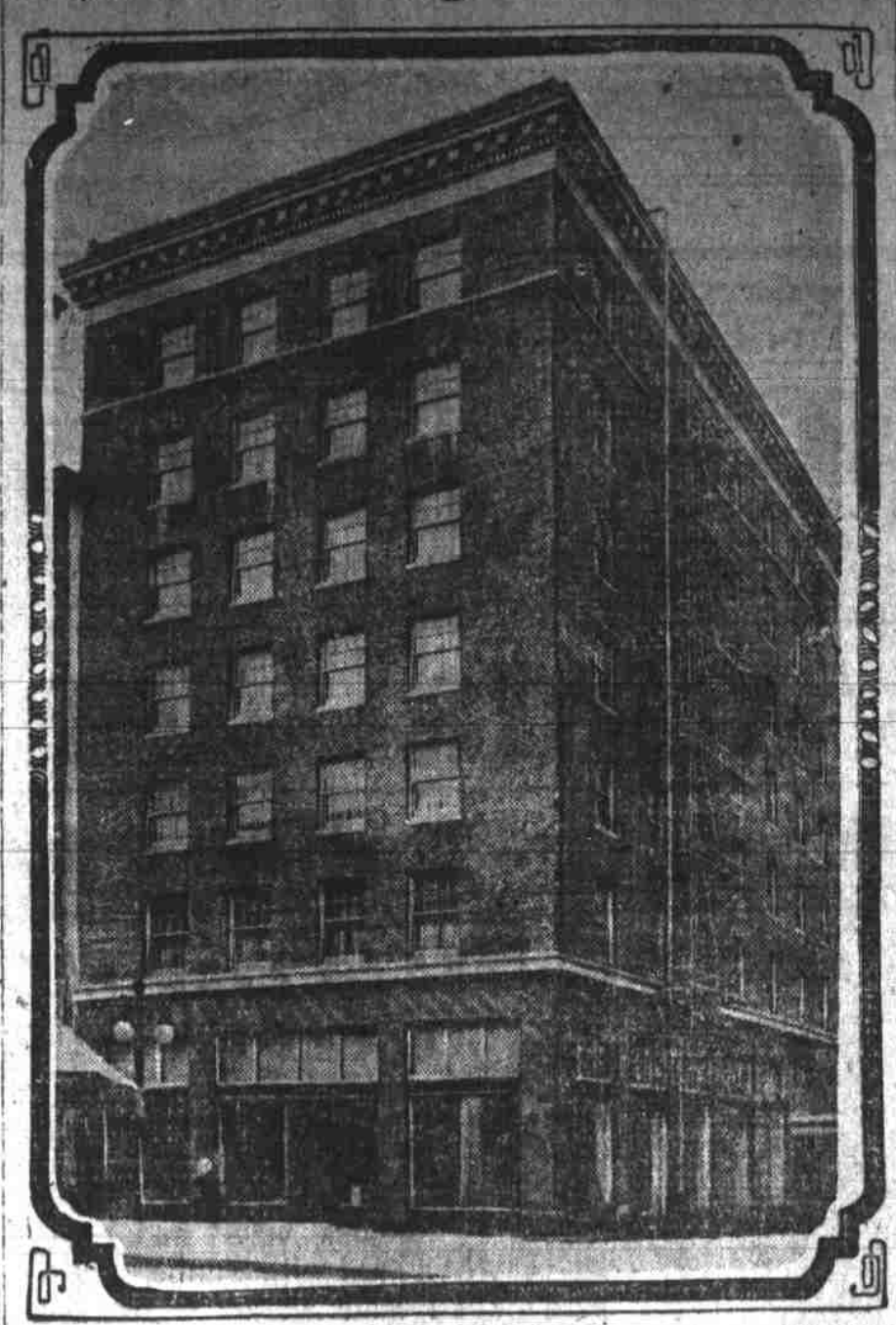
View of the recently completed Willard hotel, erected by the Shasta Investment company, at Park and Morrison streets. This is a seven story structure, which cost in the neighborhood of $150,000 and is one of the latest and most substantial improvements on Morrison street. The building was constructed to allow the addition of three more stories if needed. Hurley-Mason company were the builders and Doyle, Patterson & Beach were the architects.
