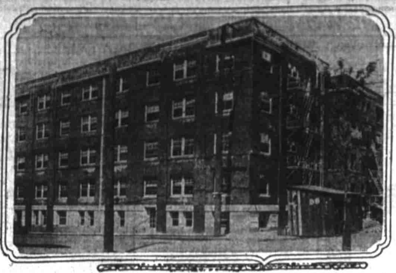
Willesley Court, four story apartment at East Fifteenth and Belmont, owned by Bailey, Taylor and Lambert. The building was recently doubled in size.
