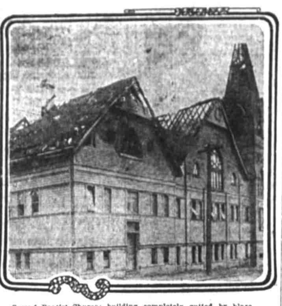
Second Baptist Church; building completely gutted by blaze.
