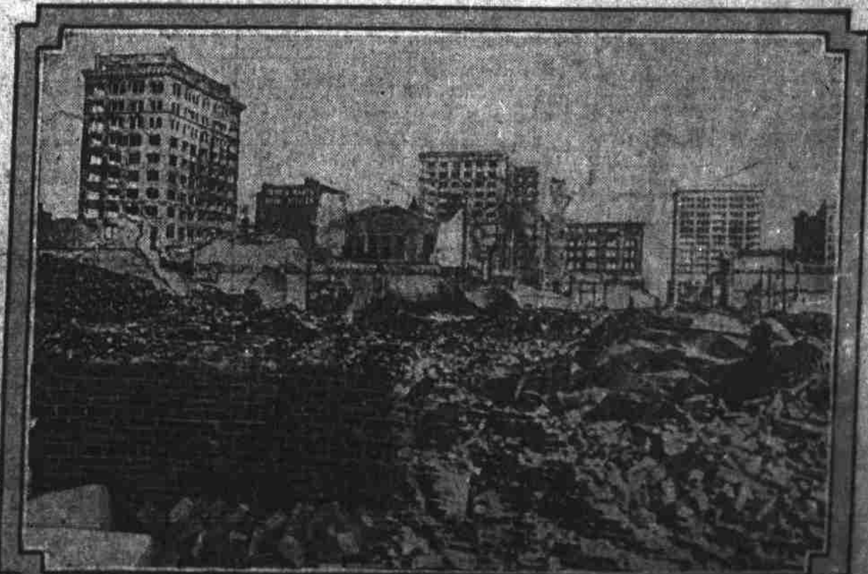
View of the Burned District of Baltimore Where Whole Blocks of Buildings Here Lost Because of Improper Window Protection.
