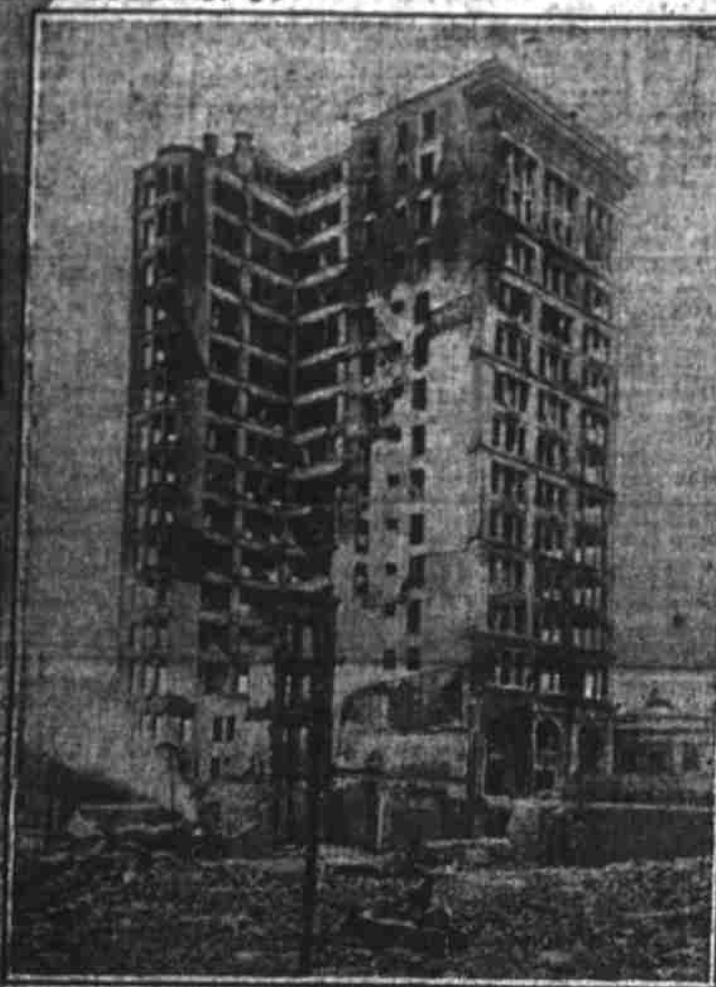
Continental Trust Company Building After the Baltimore Fire, Showing How the Structure Was Saved Because the Windows Were Not Properly Protected.
