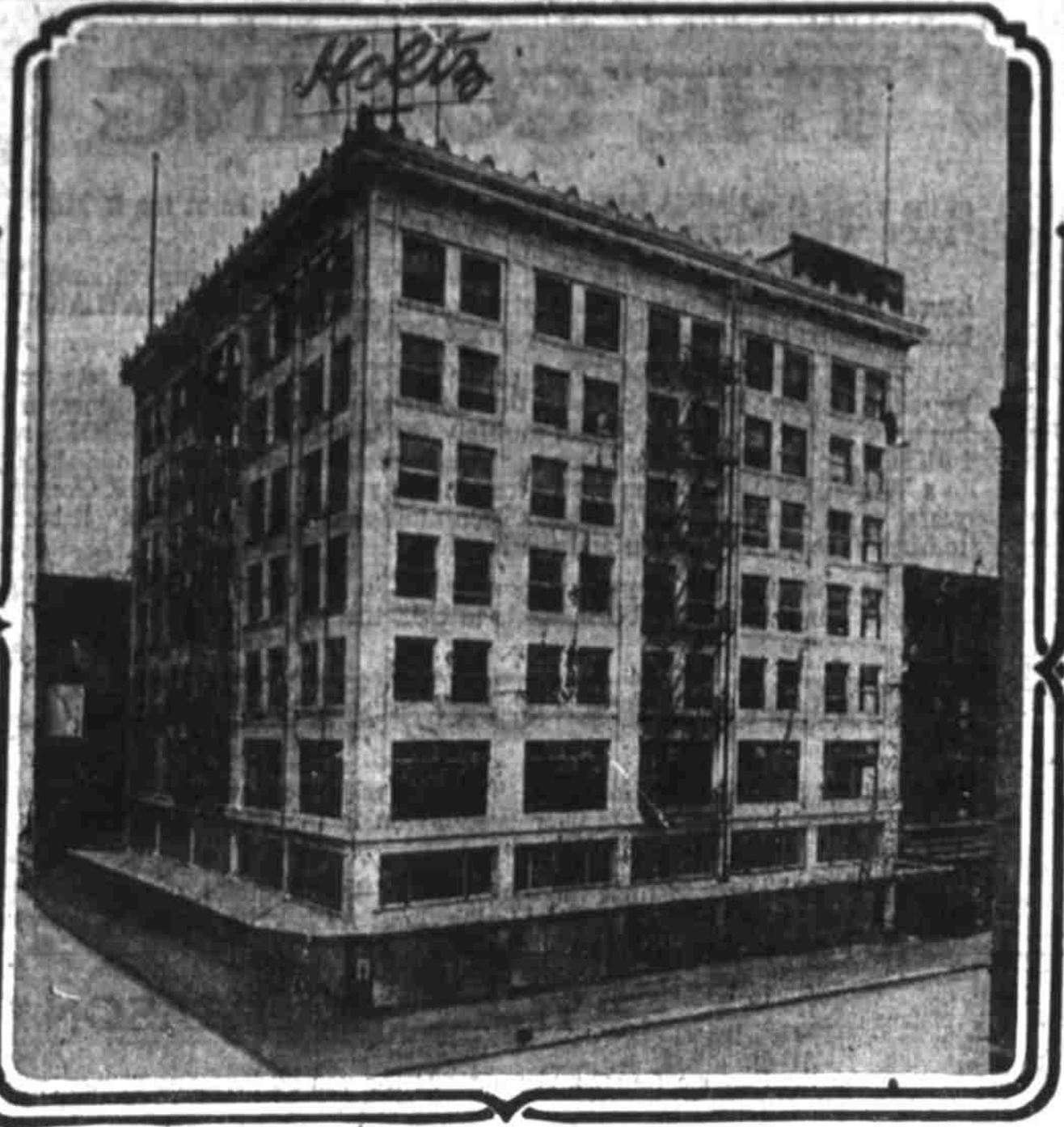
Holt's department store at Fifth and Washington streets, completed and ready for occupancy—Quickest piece of re-enforced concrete construction ever put up in Portland.
