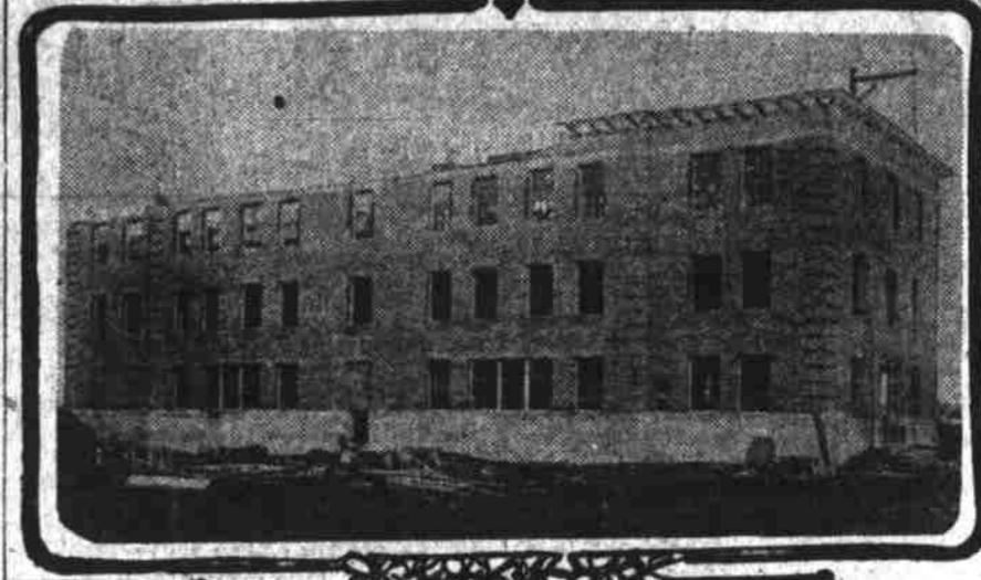
New Oregon Agricultural College Dairy building, nearing completion.
