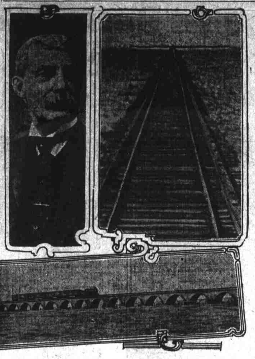
Two views of the great trans-ocean railway from Miami, Florida, to Key West, which will be formally put in service on Monday, and the originator of the epochal project, Henry M. Flagler. The upper picture shows a view along the tracks of the Long Key viaduct, which is nearly seven miles from end to end. The lower photograph gives a good idea of the manner of its construction. It has 186 arches, and is expected to stand as a marvel to engineers in the years to come. The entire length of the over-sea road is 156 miles.
