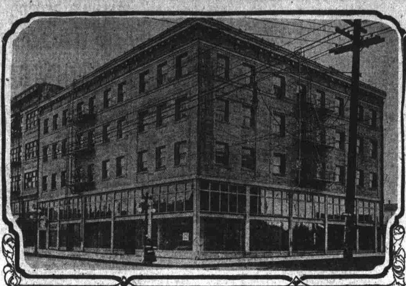
Four story store and apartments erected for Morgan, Fleidner & Boyce at East Stark street and Grand avenue.
