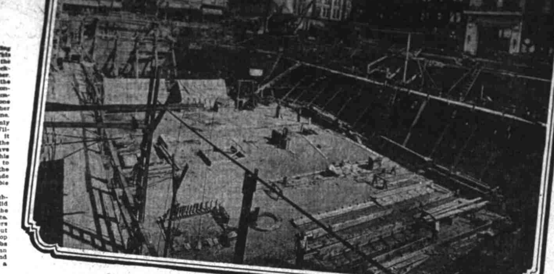
EXCAVATION NEARING COMPLETION
