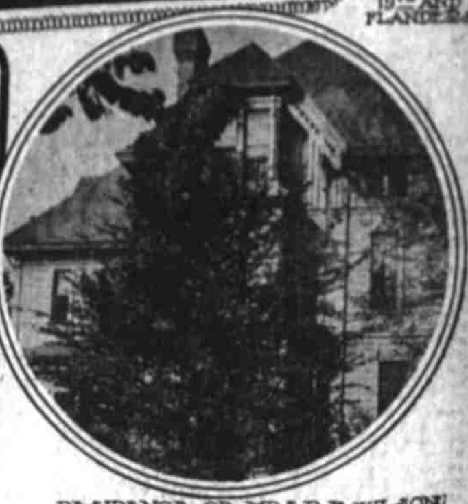
RESIDENCE OF MRS R.B. WILSON 2012 AND HOYT STS
