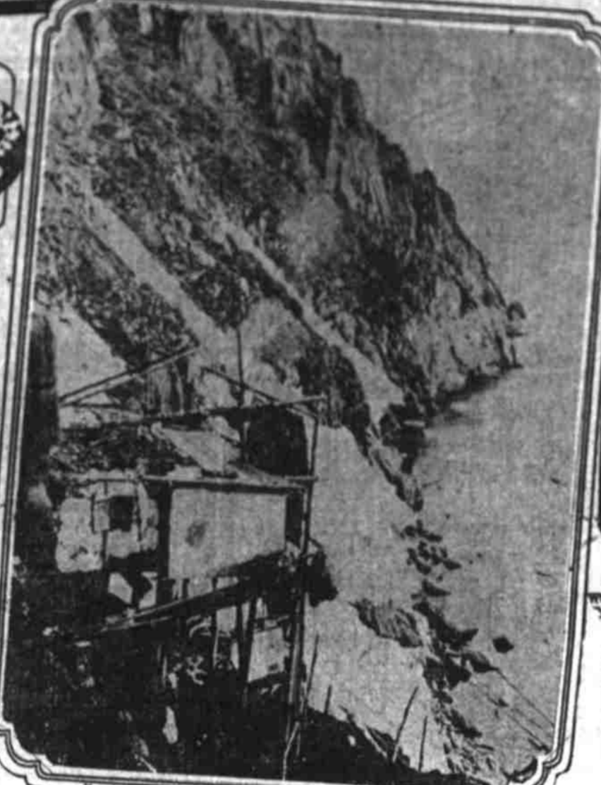
HOUSE HANGING ON SIDE OF CLIFF KING ISLAND
