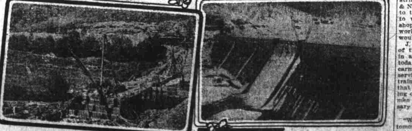
The Pulp and Paper company power dam at Austin, Pa., was built in the summer and fall of 1909. In the succeeding January, during a flood, much alarm was caused by earth slides and cracks that appeared in the face of the dam. The dam was emptied by means of a hole blown with dynamite. Nothing was done toward reinforcing the work and it was used until the catastrophe came.
