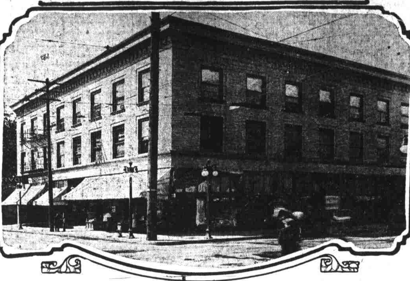
Substantial brick structure built by Ion and C. H. Lewis, on the former site of the Williams Avenue school at Williams Avenue and Russell Street, Upper Albina.
