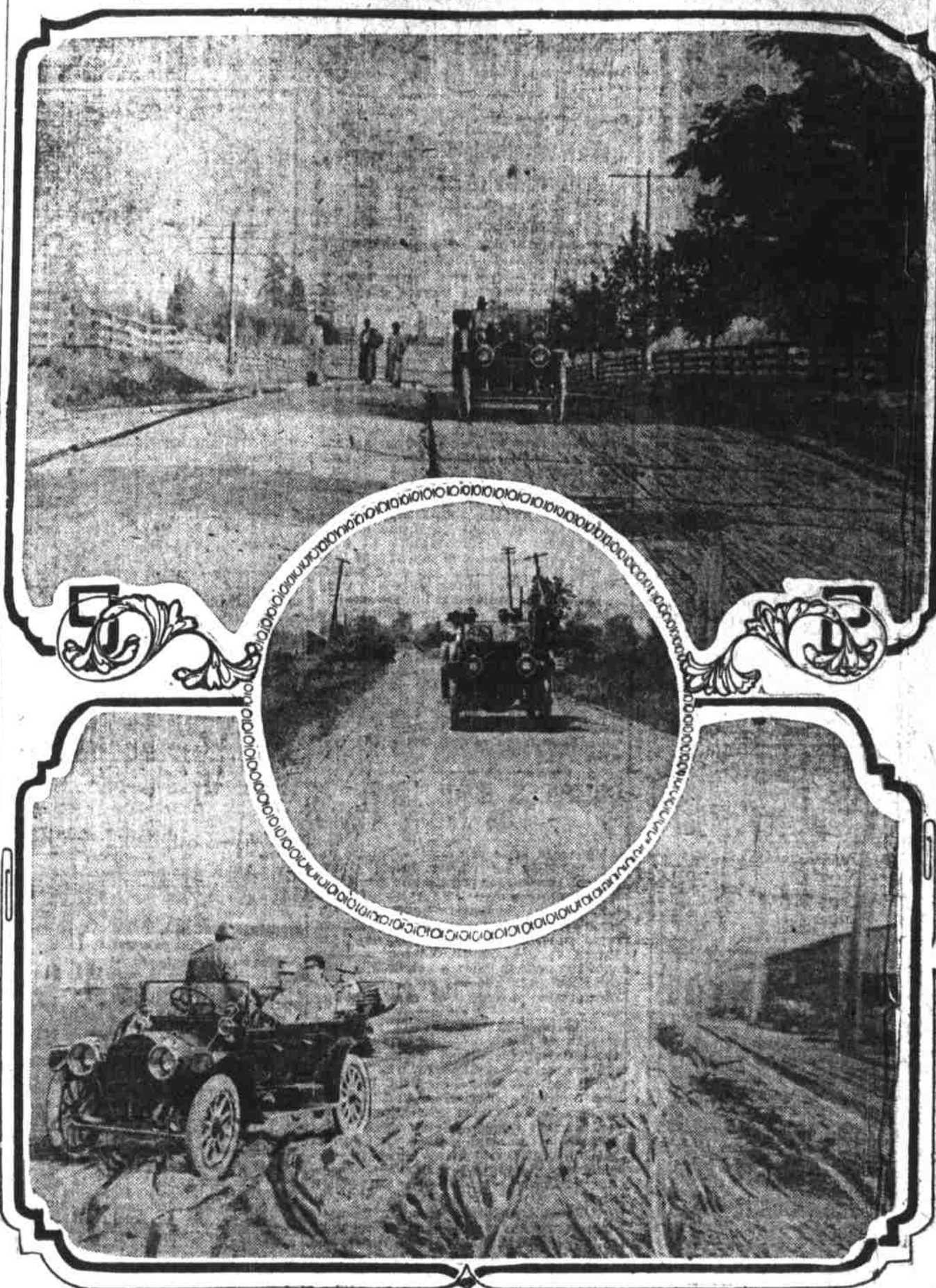
Section of excellent highway constructed by Frank Jagger in Clackamas county, south of Oregon City, on the east route of the proposed Capital Highway—But of convict built highway; Capital Highway commission members in auto, Governor West on running board—Worst section of road on entire trip found in South Portland.
