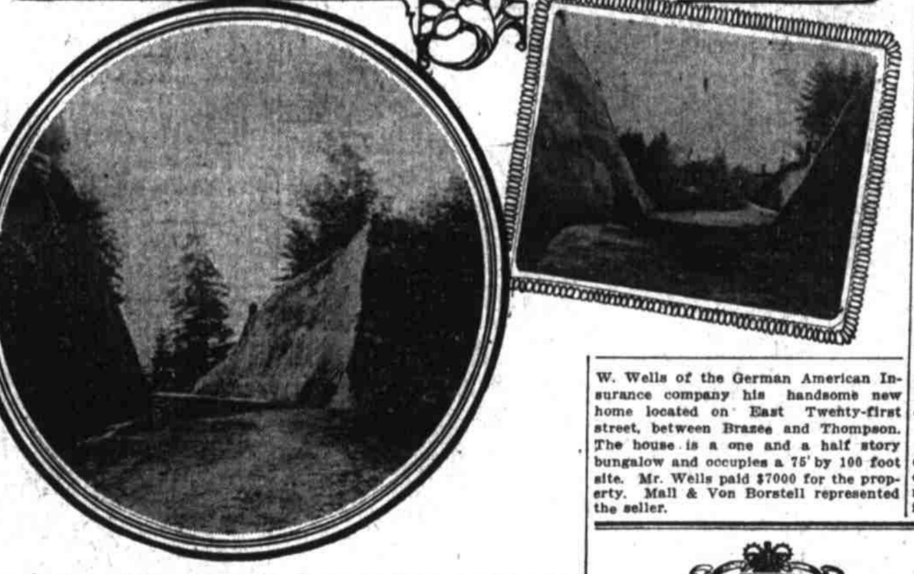
Views showing work on grade on the Clackamas Southern Railway between Oregon City and Molalla.
