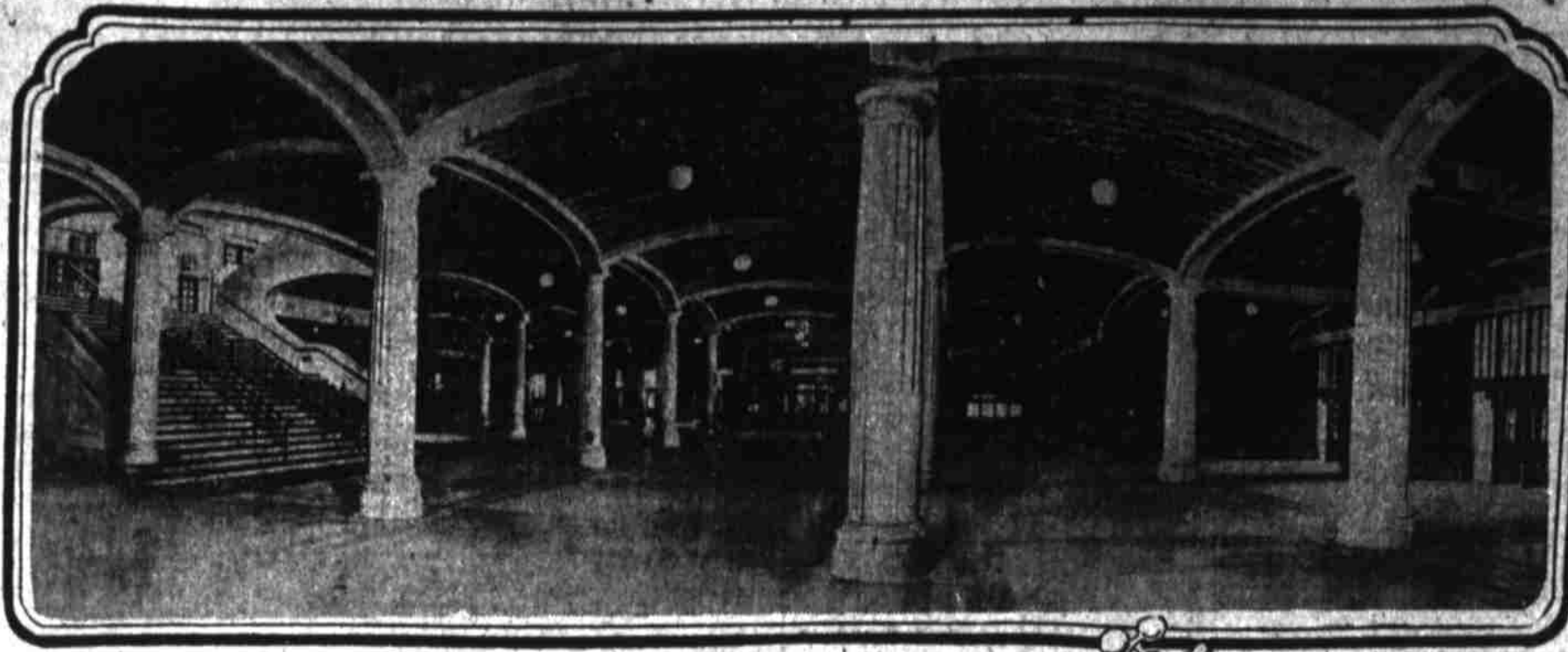
Information bureau and ticket office of the $20,000,000 depot, just completed by the Chicago & Northwestern railway.
