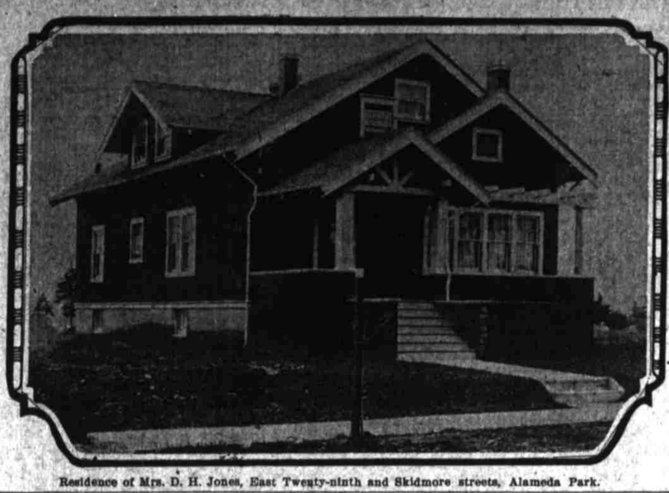
Residence of Mrs. D. H. Jones, East Twenty-ninth and Skidmore streets, Alameda Park.
