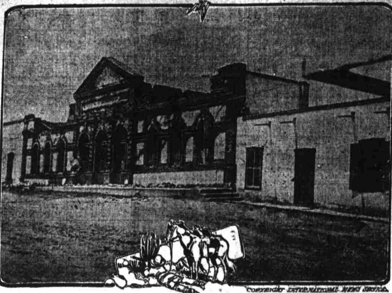
Photograph showing the havoc wrought by rebel bullets at Juarez during the battle which resulted in the capture of the city from the federalists. The picture shows the effect of a succession of volleys on a building in which the federalists were barricaded during the rebel attack.
