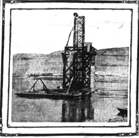
Machine lifts water 65 feet and at six turns a minute a ten inch pipe with four foot head could not take care of the flow. The machine will discharge 3000 gallons a minute at 22 revolutions.
