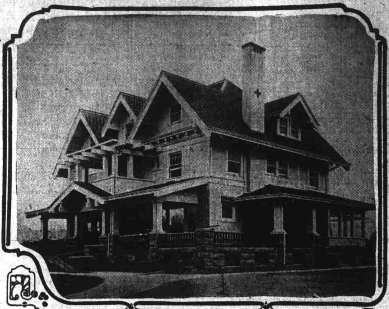
Fourteen room dwelling under construction for Andrew R. Porter.
