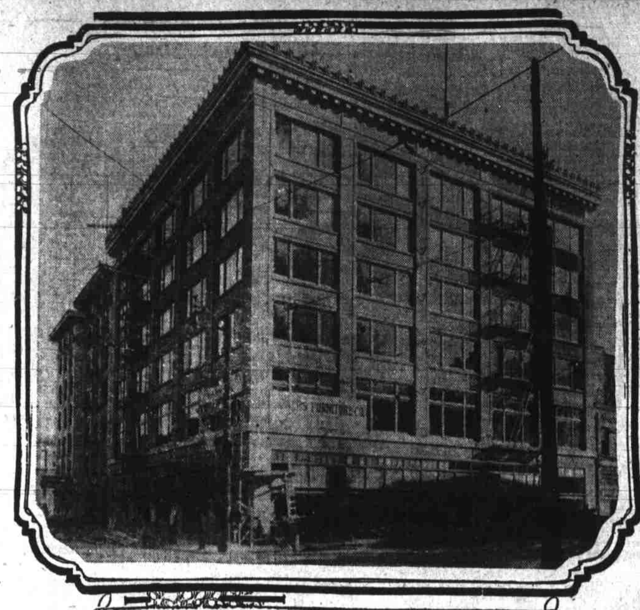
New home of Powers' Furniture Company, at Third and Yamhill; building is practically completed and will be occupied about April 1.
