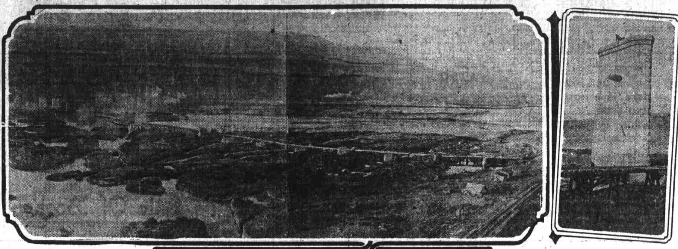
Fine structure is to be 3800 feet long and will be ready early in summer.
