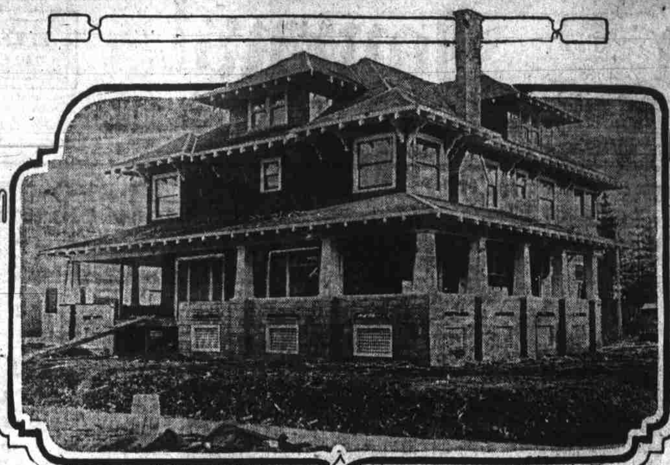
Remains of L. T. Wilcox, under construction at East Twenty-first and Braze streets.
