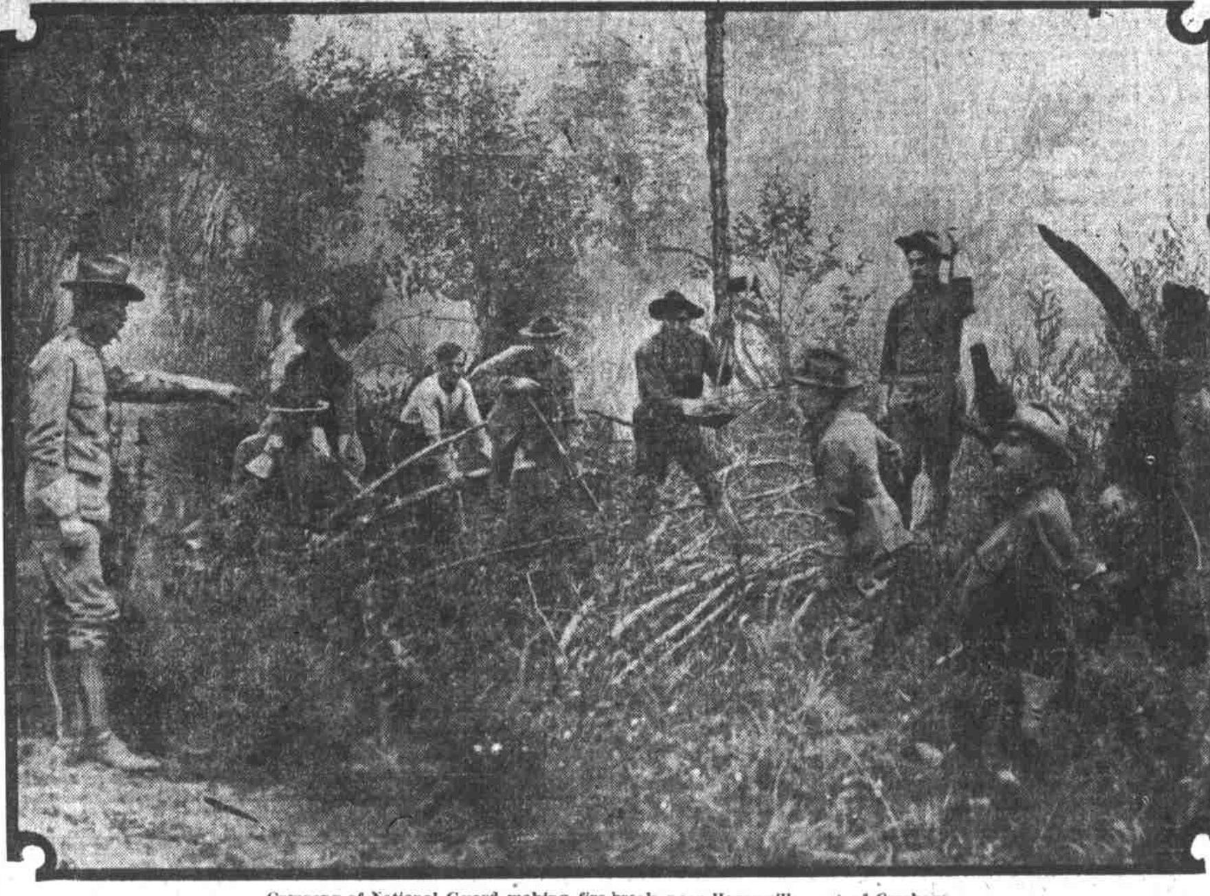
Company of National Guard making fire-break near Hoganville, east of Gresham.
