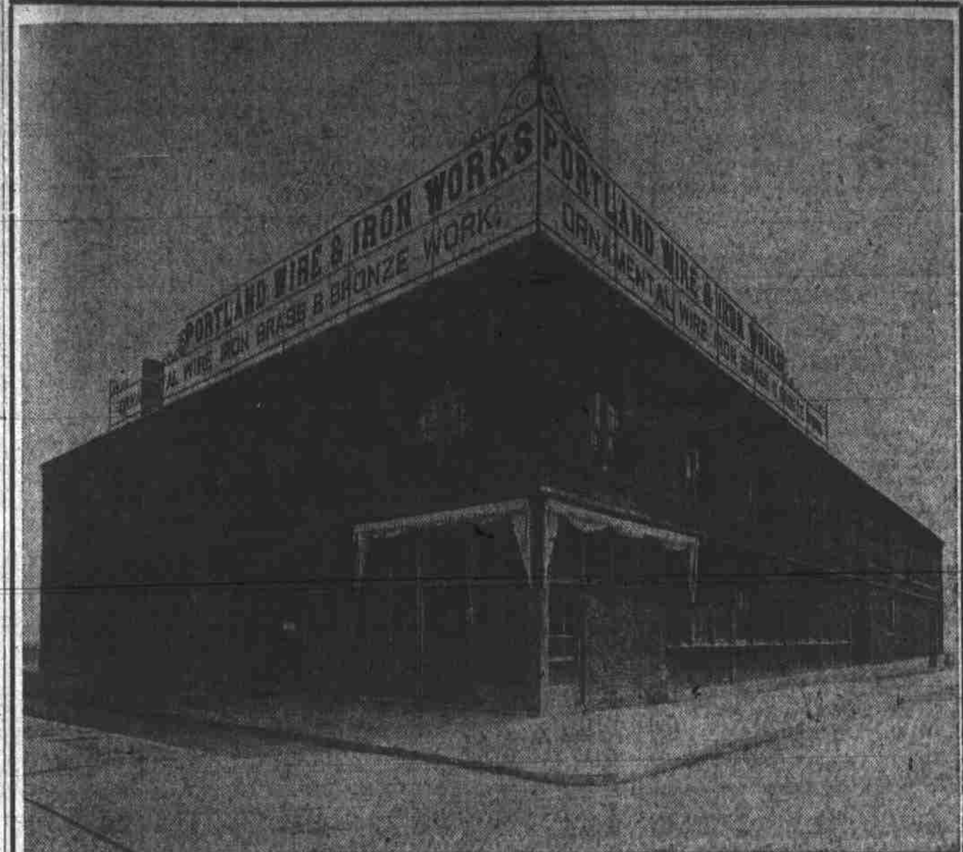
This substantial structure just completed at Second and Columbia streets. Now the permanent location of the Portland Wire and Iron Works, coast leaders in Ornamental Iron Work
