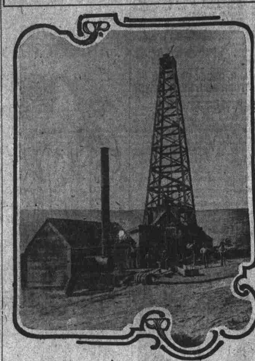
Drilling outfit at the Eastern Oregon Oil company's well.
