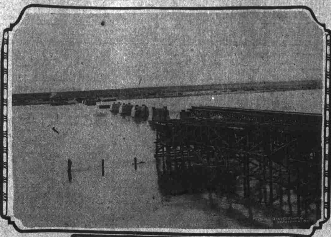
North Coast railroad bridge under construction. Nine concrete piers finished.
