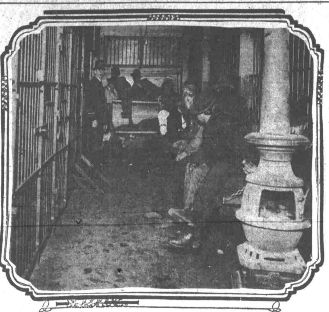
Flashlight picture showing interior of the "drunk" cell.
