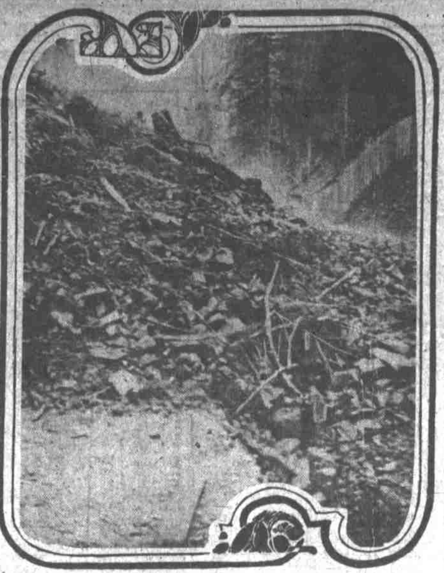
Huge pile of rock dislodged as the result of a blast fired at the Linton rock quarry Saturday when four tons of powder were used. Enough material was dislodged to keep city prisoners busy for a year.
