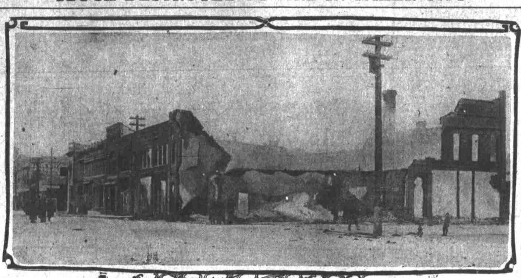
Photograph Taken for The Journal, Showing Damage Done by Flames to Prominent Business Block of Baker.
