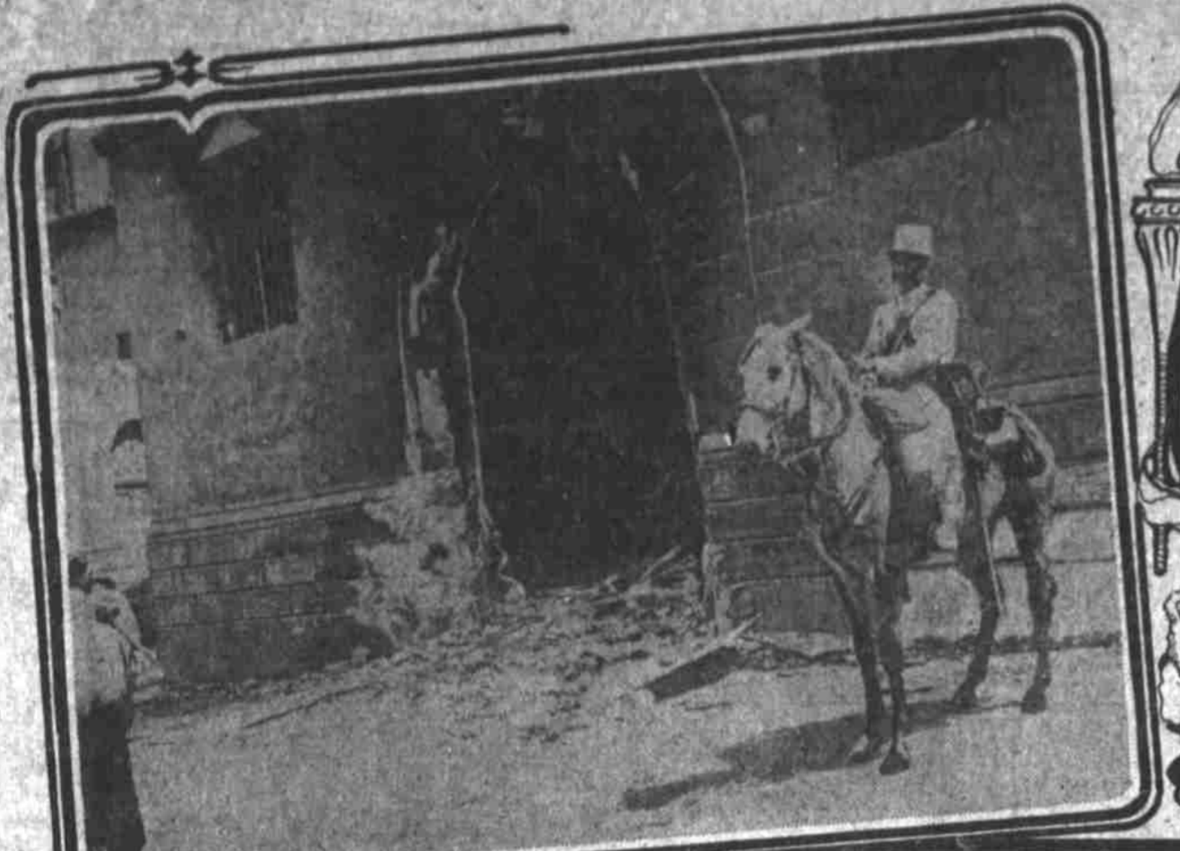
FACTORY DOORWAY DAMAGED BY BARCELONA BOMBS.
