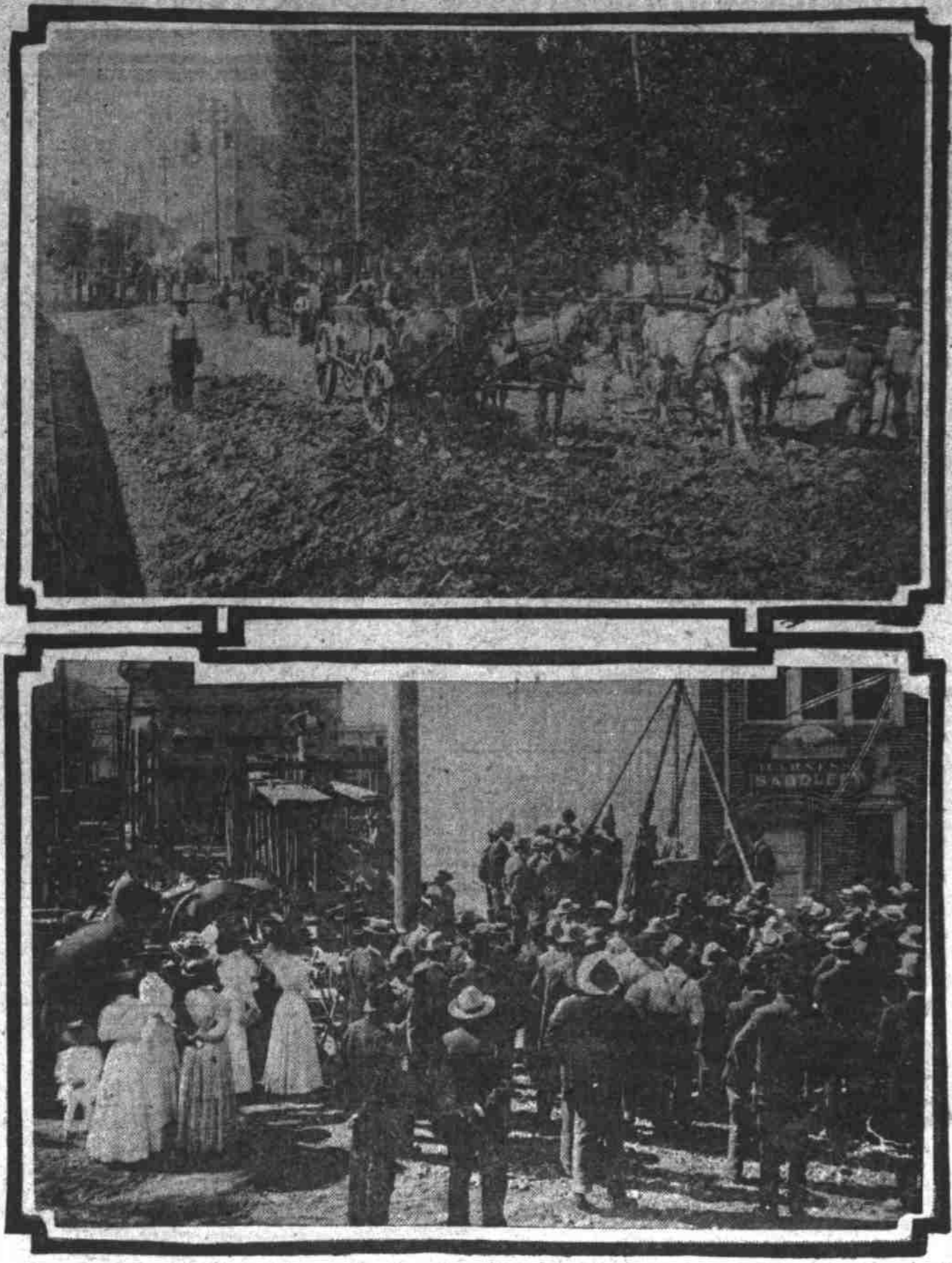
Paving crew at work near courthouse. Laying cornerstone of brick block.
