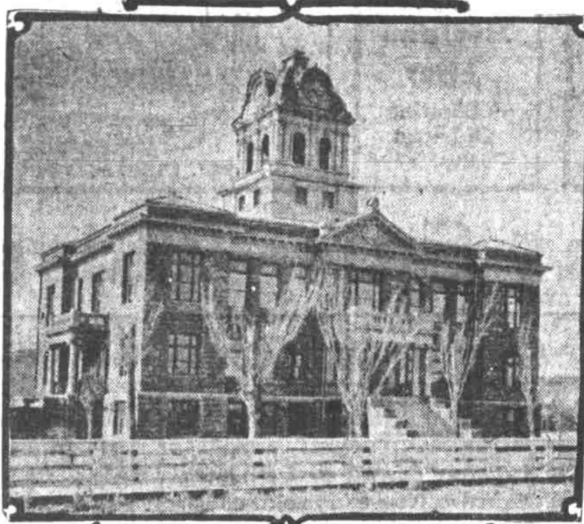
New Courthouse of Crook County. Just Completed at Prineville.
