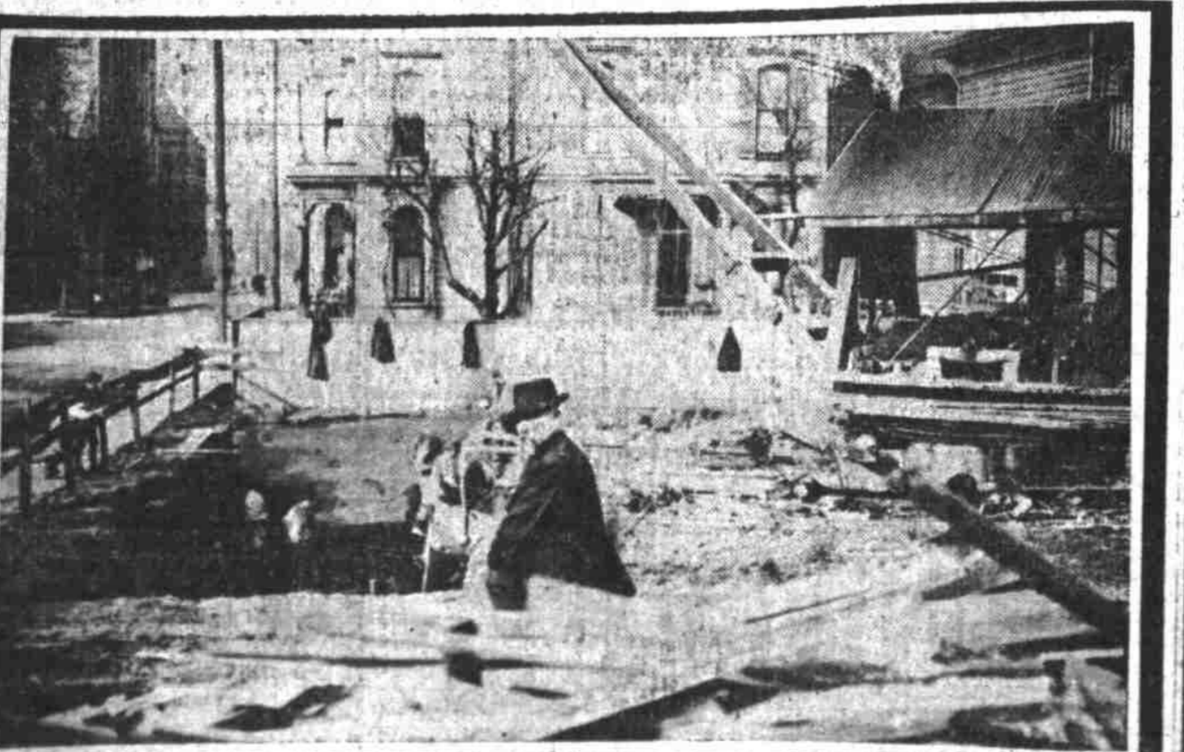
Breaking Ground for New Arlington Club Building, Salmon and Park Streets.
