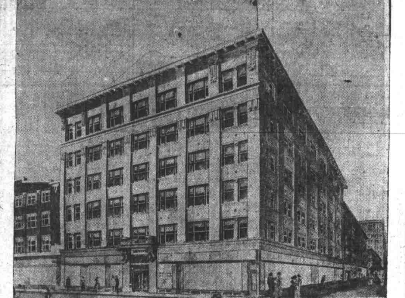
Charles K. Henry Building, Under Construction, at Fourth and Oak.
