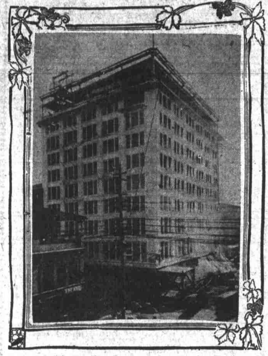
Meier & Frank Building, Under Construction at Sixth and Alder Streets.
