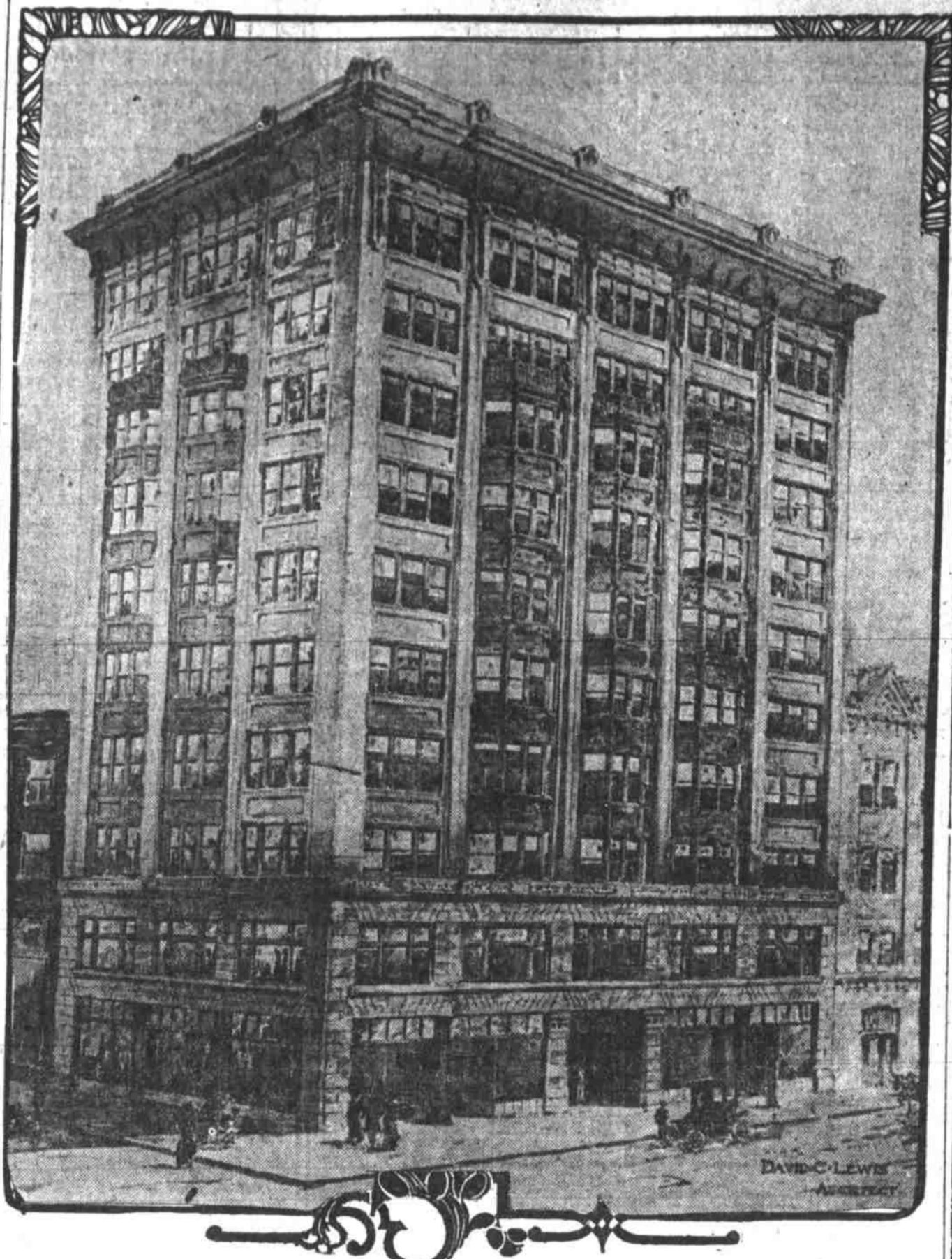
Lewis Building Under Construction at Fourth and Oak Streets.
