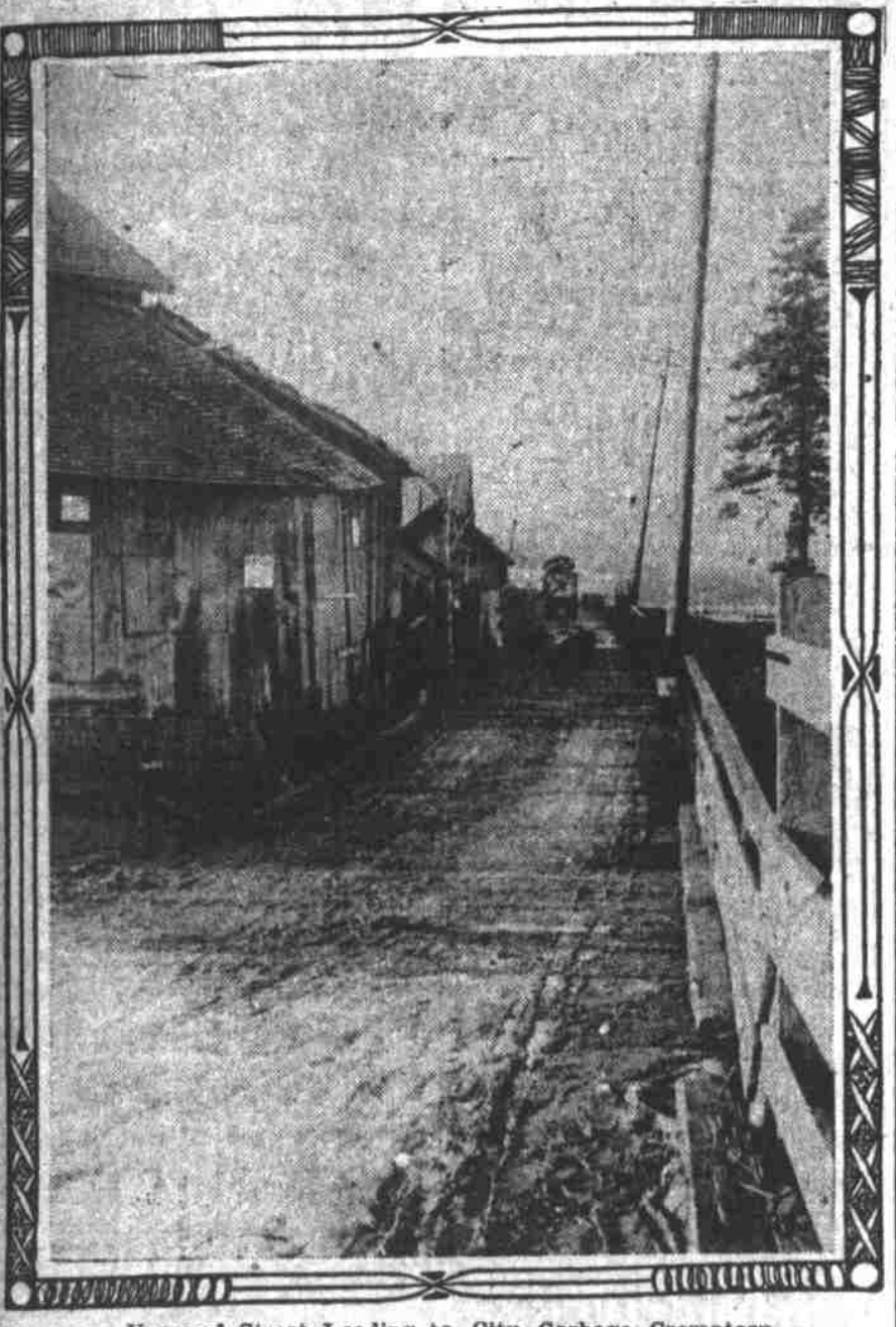
Unpaved Street Leading to City Garbage Crematory.
