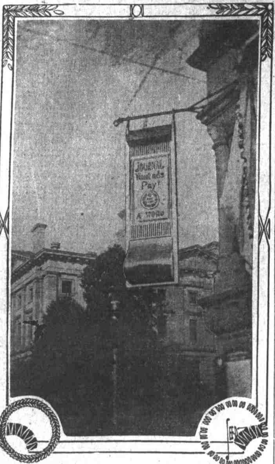
Journal Chimes Just Installed at Fifth and Yamhill Streets.
