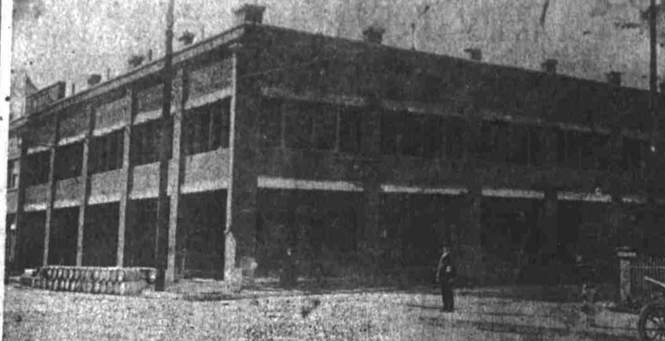
New Wemme Garage, Seventh and Burnside.
