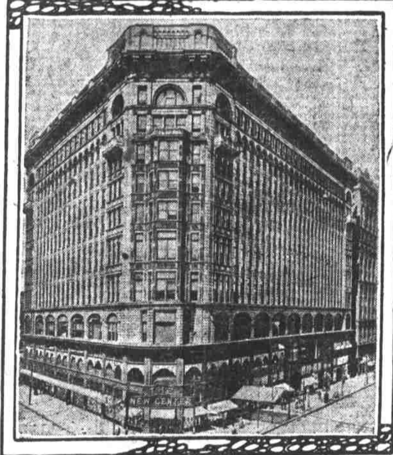
Rose Building, Cleveland, Part of the Estate
