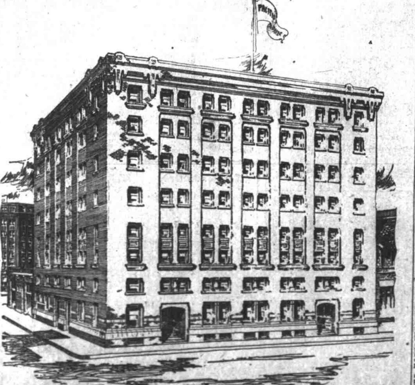
The new building of the Pacific Paper Company under construction at Fourth and Ankeny streets will be one of the best equipped commercial buildings in the city. It will be six stories high, with a steel frame and concrete walls. The building will be equipped with the most modern and approved fire protection sprinkling system. Two electric elevators are to be installed. The building will be completed and ready for occupancy by February 1, and will cost about $70,000.
