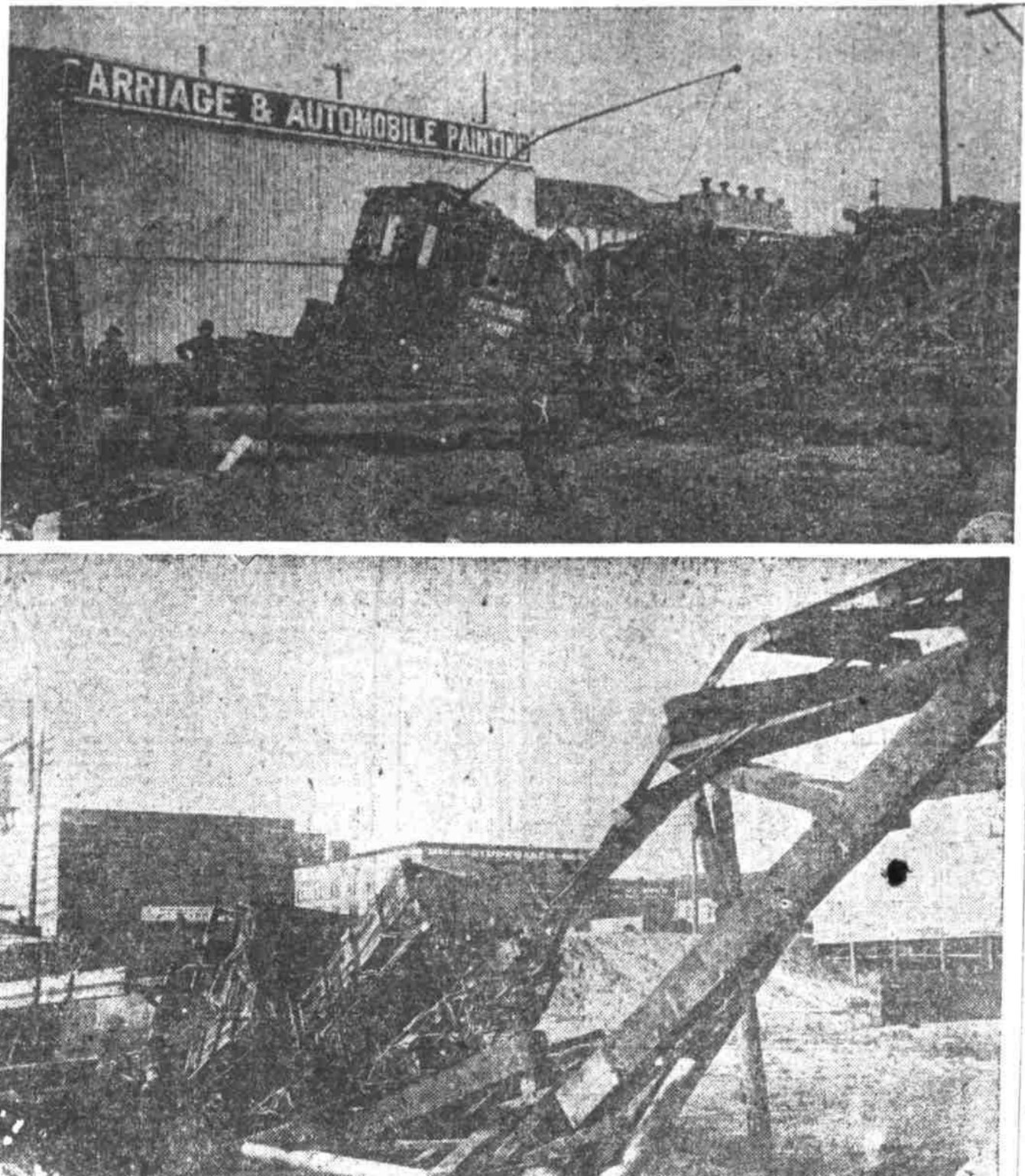
Gravel Train and Trestle Wrecked on East Side Hill.
