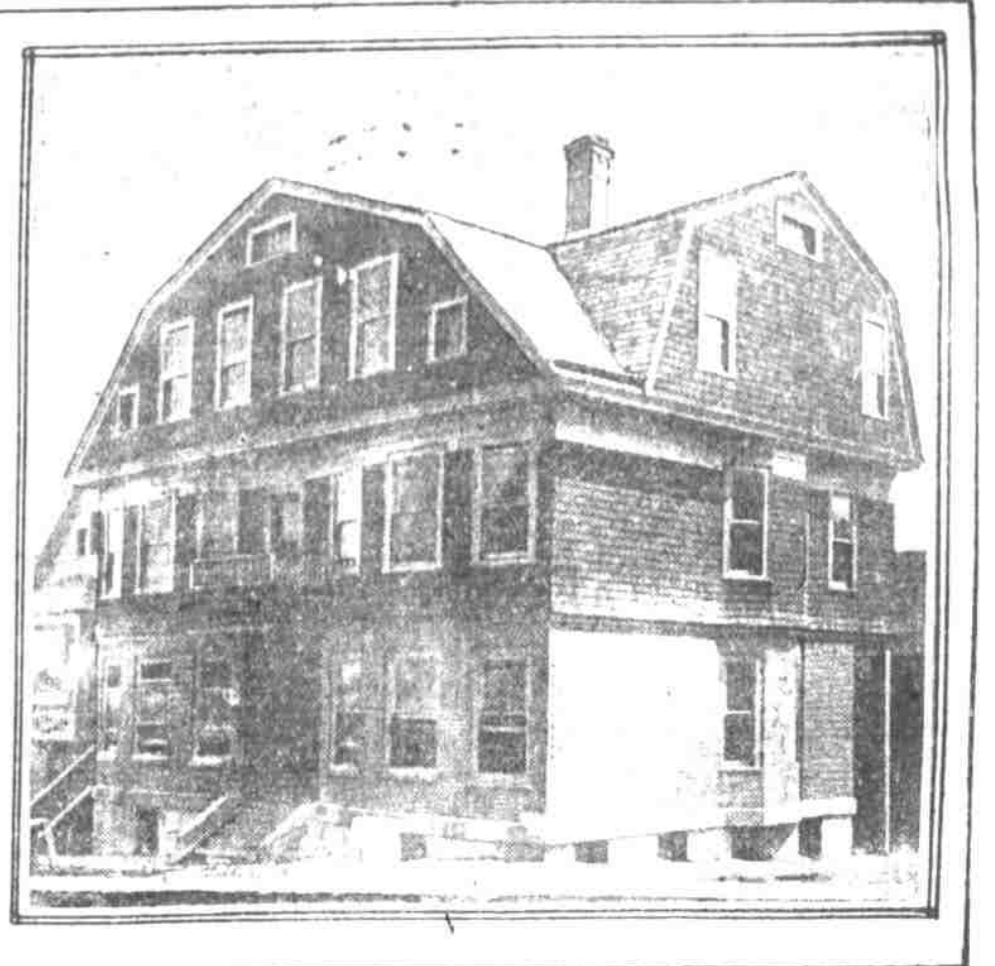
Apartment House, Dunham Investment Company, Eleventh and Jackson Streets.
