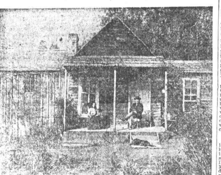
Home of J. L. Porter, on Rice Creek, in Douglas County—Typical Pioneer Homestead of Southern Oregon.
