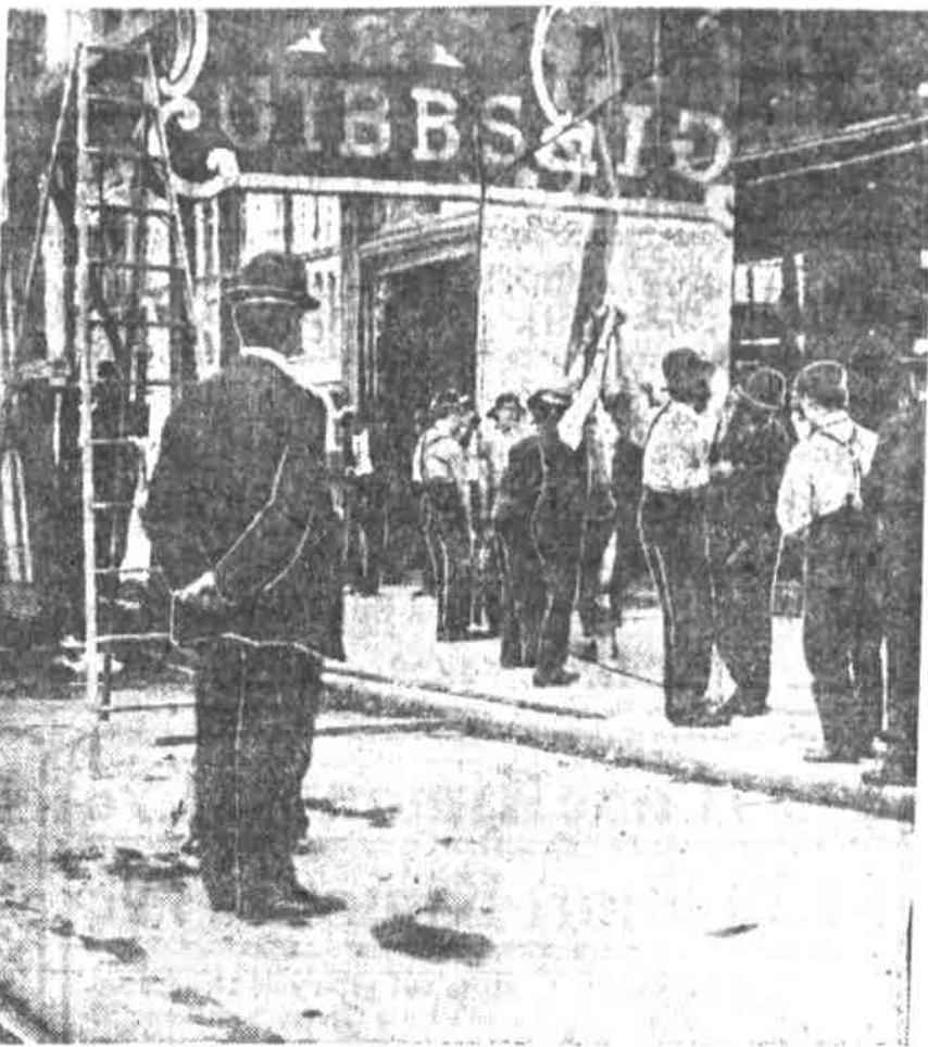
Eight Men Required to Handle Plate 10x15 Feet and Weighing 700 Pounds. Settling of Building is Supposed to Have Broken the Original.
