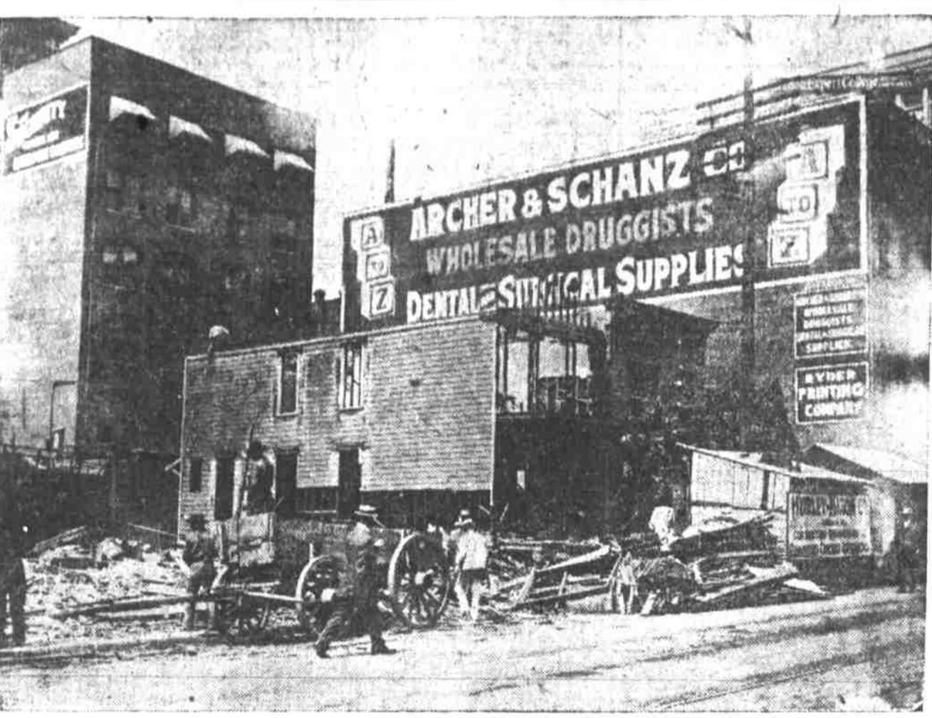
Site of Lombard Building, at Fifth and Stark Streets.
