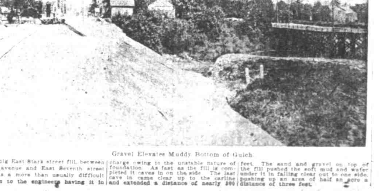
Gravel Elevates Muddy Bottom of Guich. The big East Stark street fill, between Grand avenue and East Seventh street, presents a more than usually difficult problem to the engineers having it in charge owing to the unstable nature of feet. The sand and gravel on top of the fill pushed the soft mud and water under it in falling clear out to one side, pushing up an area of half an acre and extended a distance of nearly 300 feet.
